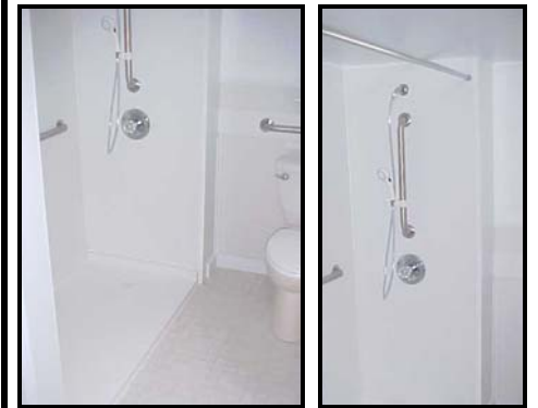
Above: A recently completed bathroom modification included the installation of a roll-in shower, an accessible sink, and grab bars around the toilet.
